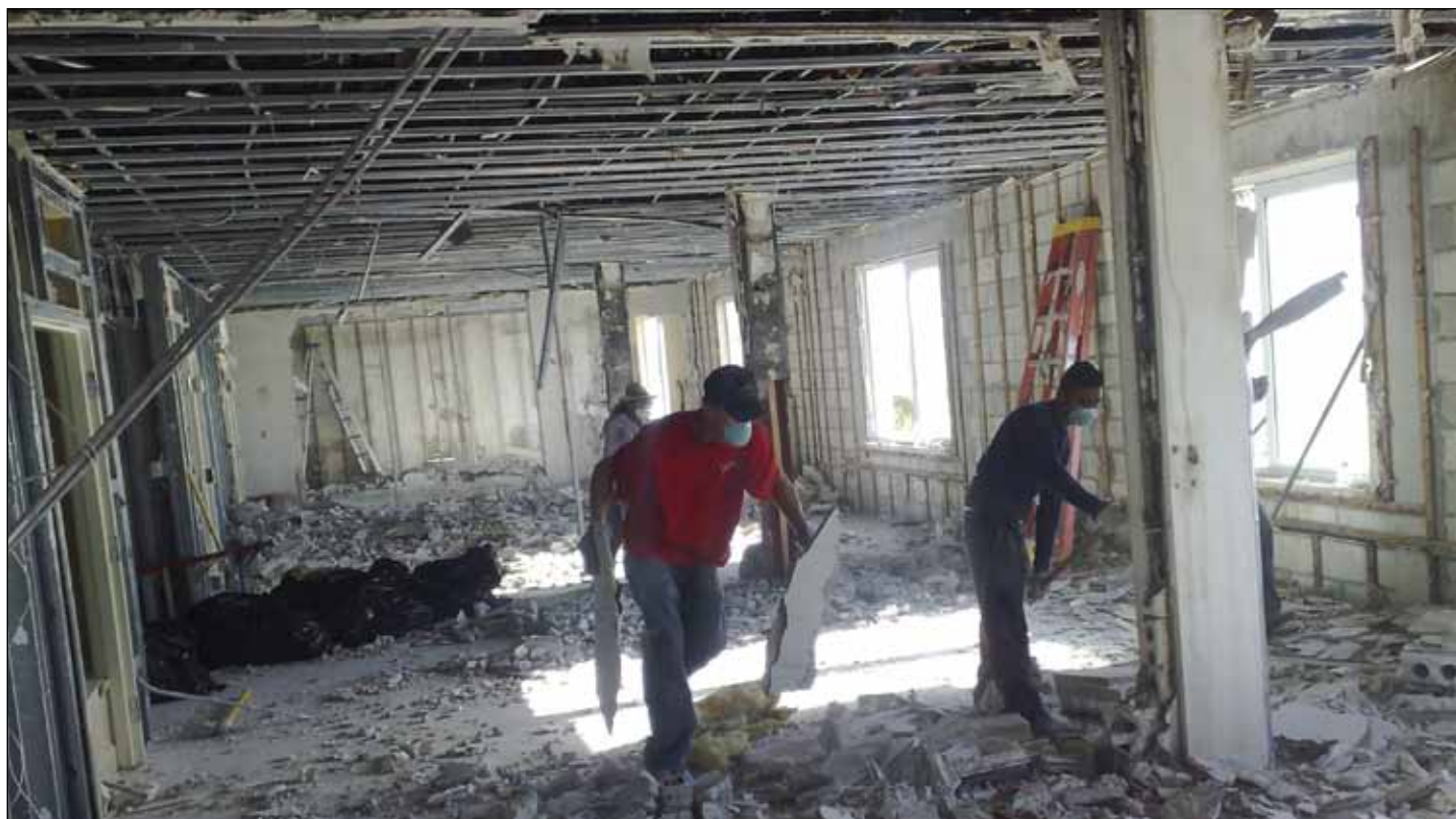
An extreme case — the main goal of Servicemaster water damage restoration is to salvage as much as possible in the way of walls, flooring and carpet, but after severe damage, sometimes it's necessary to rip out drywall to the bare studs, as was done on this demolition site.
