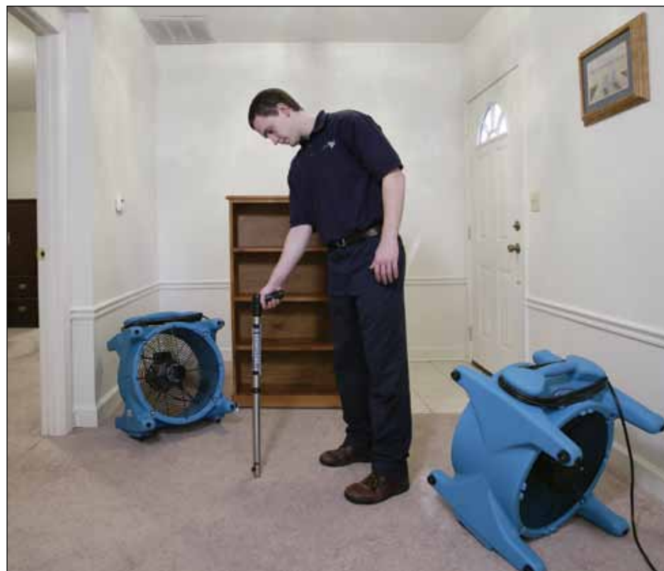
Technicians use high-velocity air movers to help accelerate the drying process and moisture monitors to monitor progress.
