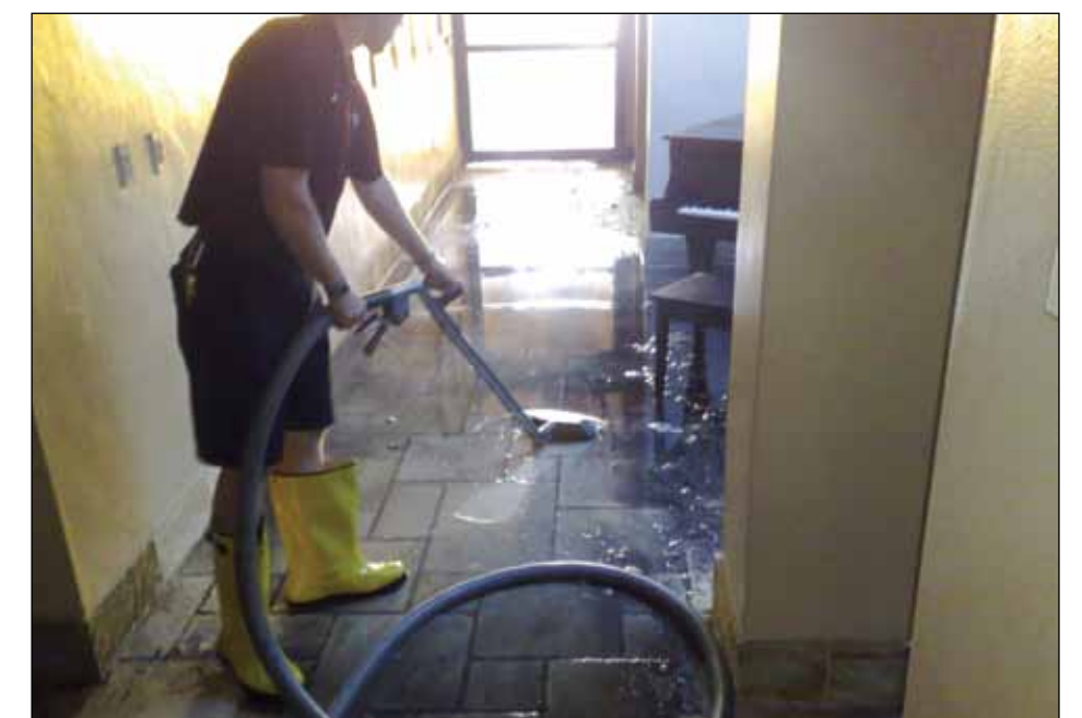
One of the first steps to water damage restoration is getting rid of any standing water using a self-contained, high-powered water extractor to suck water from floors, walls and baseboards.
